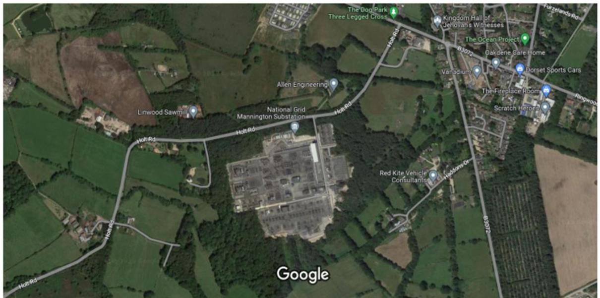
Plate 3.1 - Aerial View of Mannington 400kV substation
